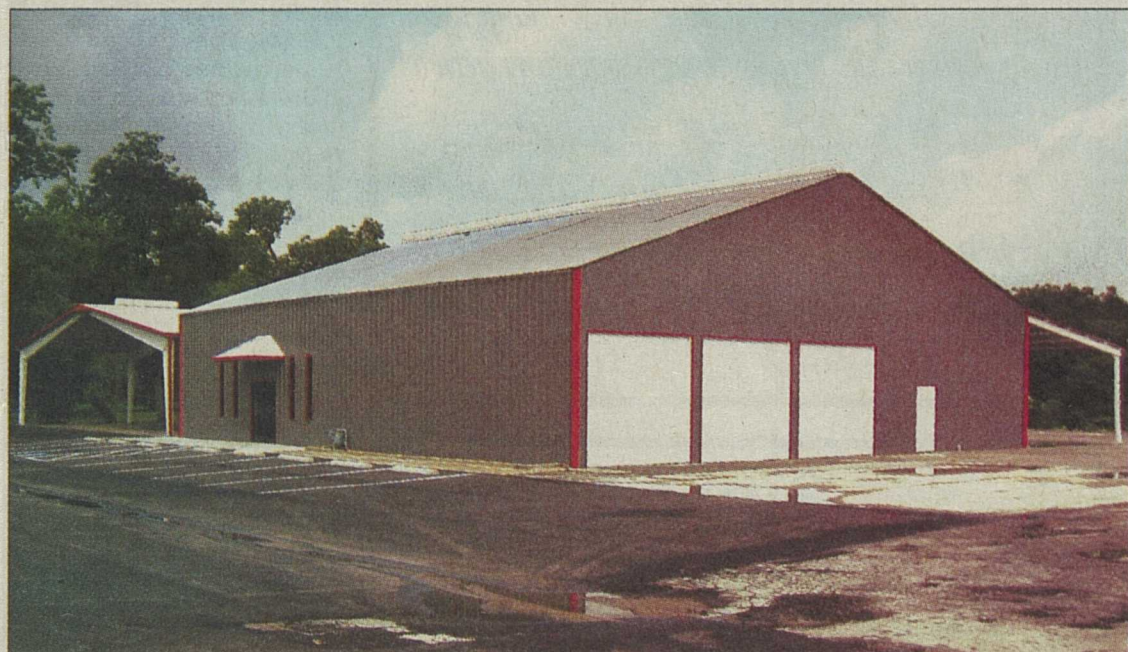
The old Lake Motors Building at 323 S. McCarty has undergone a $160,000 renovation and will re-open in late July as a new location for Purvis Industries.
